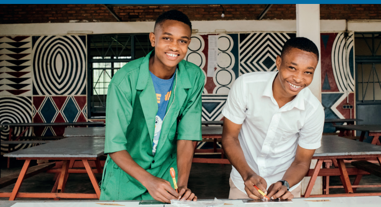
Even the teenagers are helping with the construction of the school.
